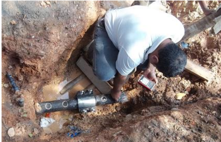
Figure 15 : Measuring thickness of 3” dia Live cast iron line
