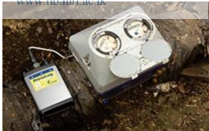
Figure 02 : Measuring Pressure of 3" dia Live cast iron line
