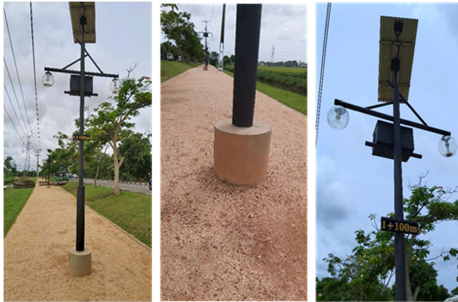
Figure 11: Landscape lighting, position, mounting method and the used materials for the lamp post in Kimbulawela Jogging track Source: author
