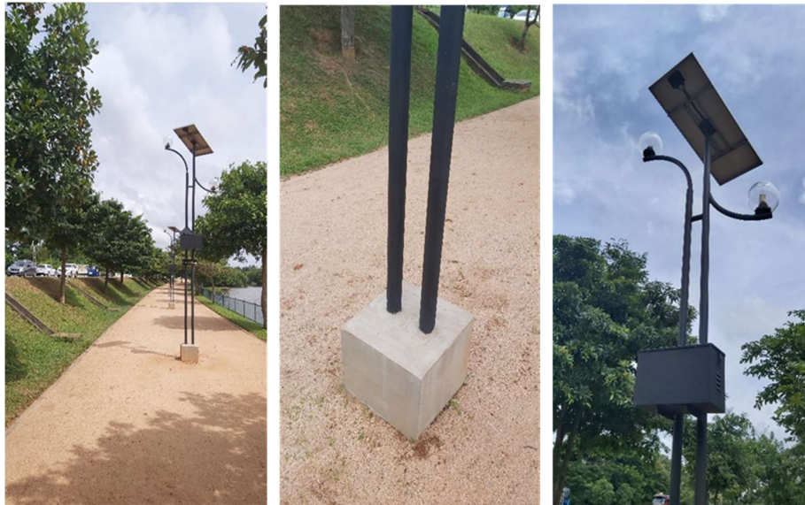
Figure 10: Landscape lighting, location, mounting method and the used materials for the lamp post in Diyawanna oya Jogging track
